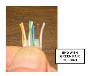
Make sure that the wire aligner is tight to the cable jacket. Untwist the wire back to the top of the wire aligner. Straighten the exposed wires as flat as possible.
